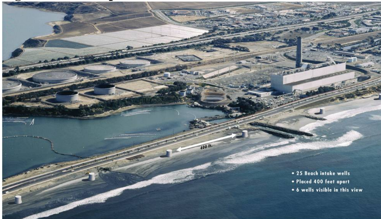
Figure 4-3 – Pump Stations with Horizontal Intakes
